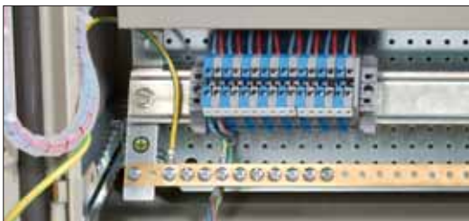
Combined fastening leg for earth collector
