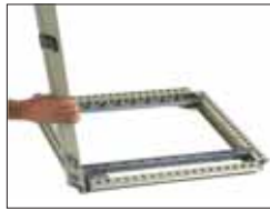
Fixing the 4 uprights to the lower and upper frames.
