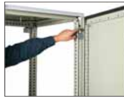
Fitting the door by fixing with studs and hinges.
